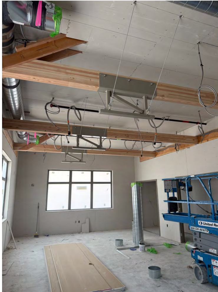
Fig. 2) Sensory gym framing and bracing for interior swings.
