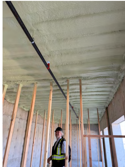
Fig. 1) Basement storage rooms.
