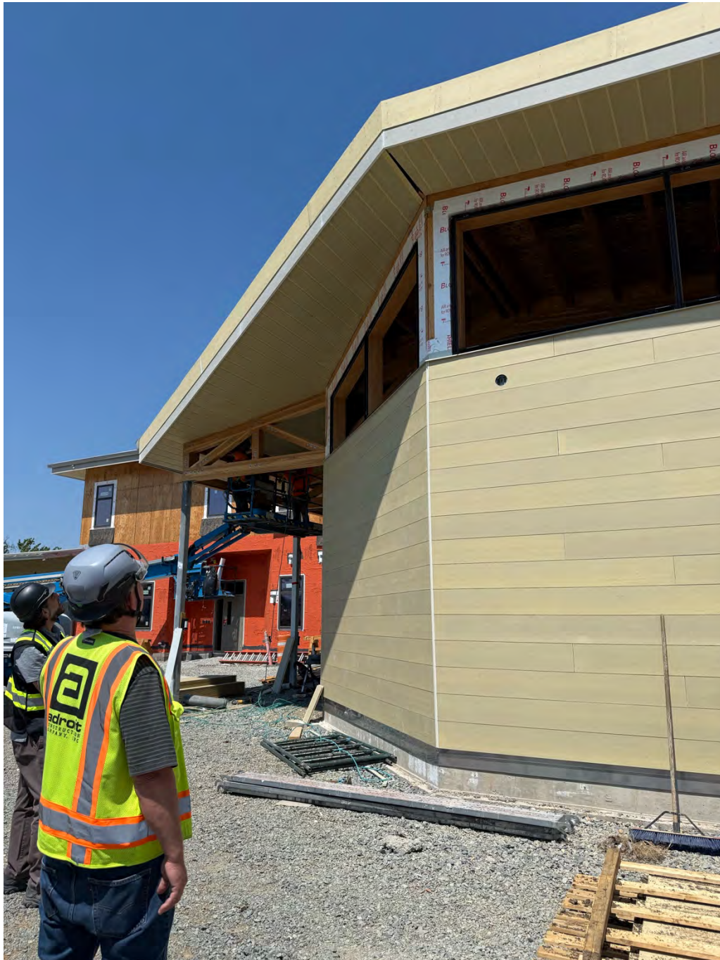
Fig. 4) Siding install complete at the front conference room.
